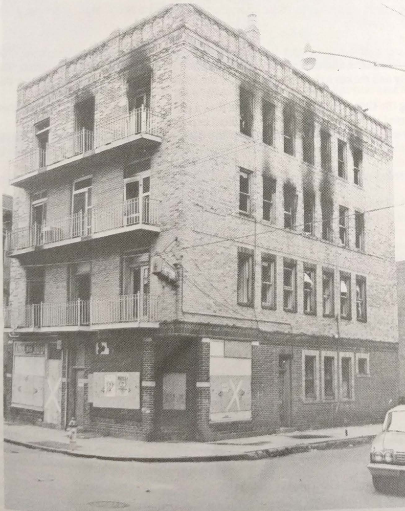
Vandalism amounts to destruction of property, including plumbing and electrical fixtures.
