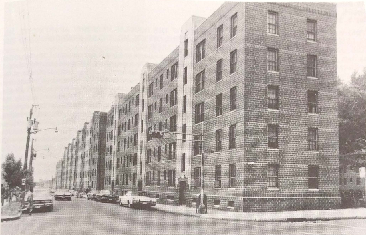
Viewing section of Douglass-Harrison Apts., cor. Spruce and Somerset Streets looking south.
